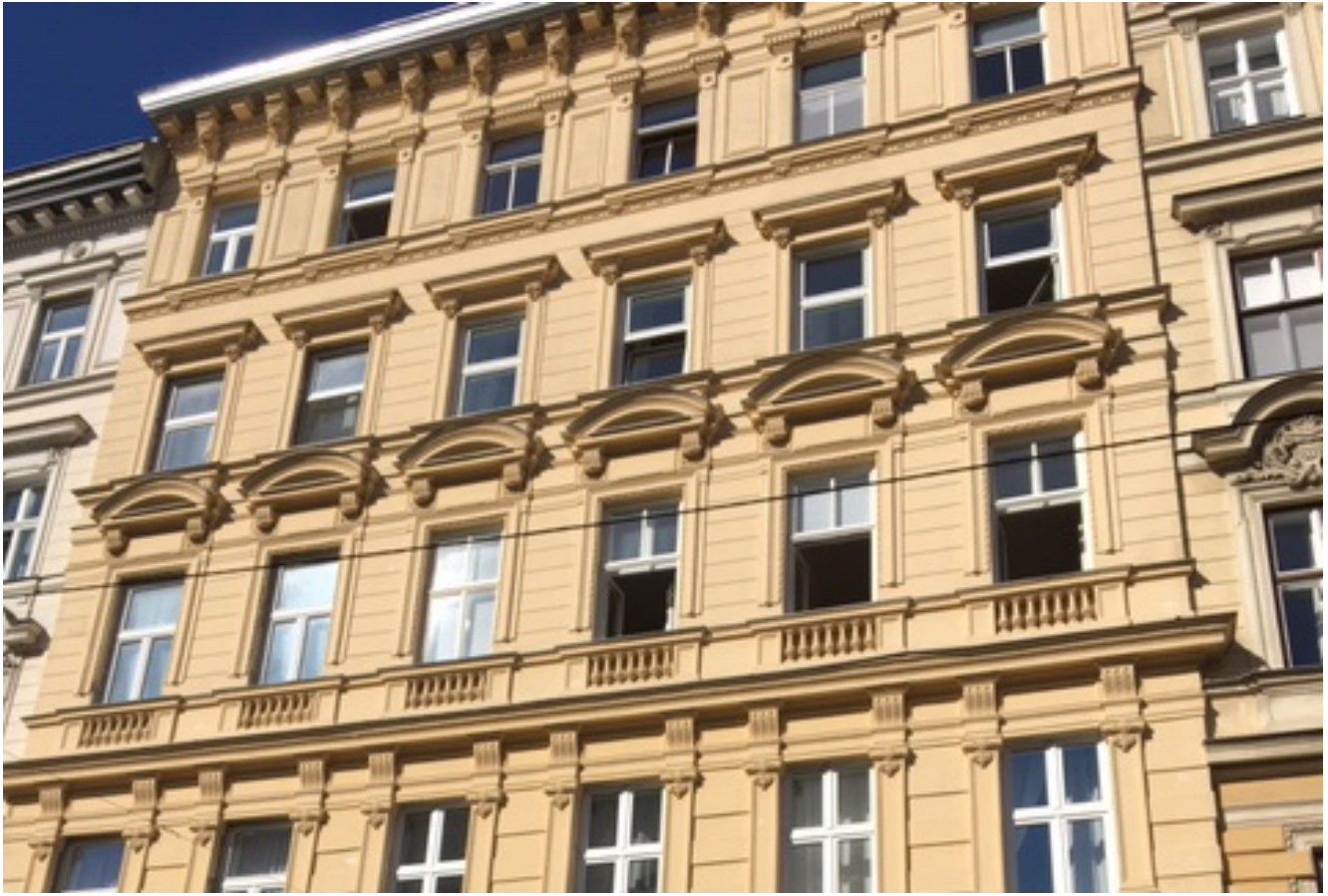
Exterior of the residence in Vienna Photo: Kultur Kontakt Austria
