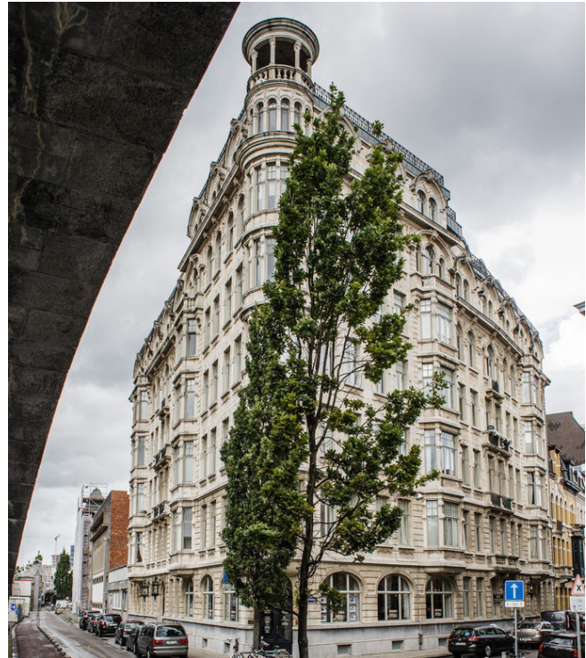
Exterior of Translators' House Antwerp Photo: Bob van Mol
